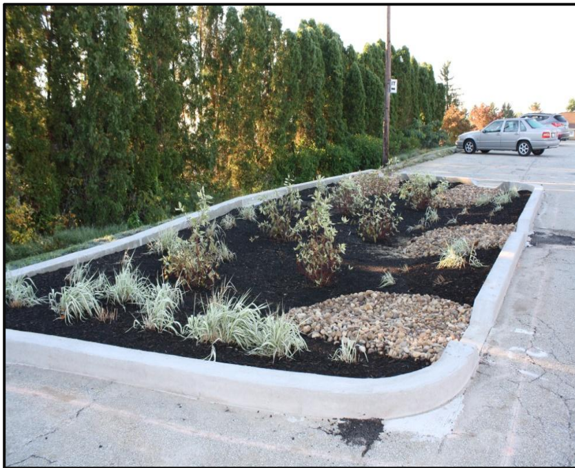
Figure 9: A rain garden in a parking lot to capture stormwater from an impervious parking lot (Source: Westmoreland Conservation District)
