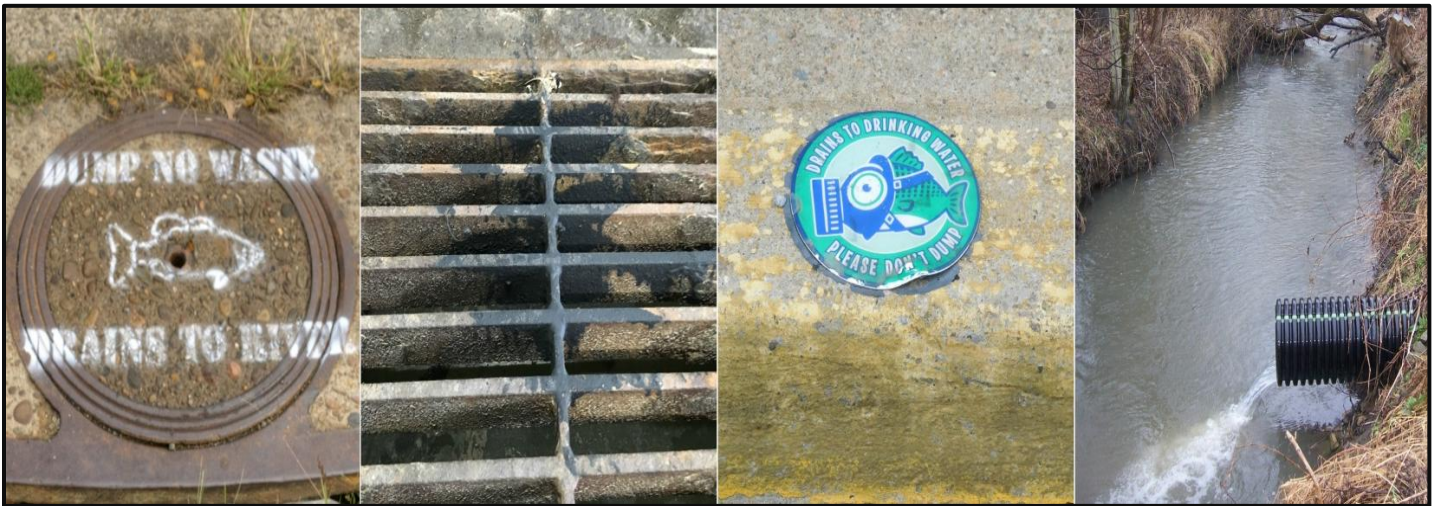
Figure 6: From left to right: A stenciled storm drain in Pittsburgh; Staining which shows some sort of illicit discharge poured down a drain; A "no dumping" stormwater identification marker in Etna; An outfall to a stream (Sources: SPC and Westmoreland Conservation District)
